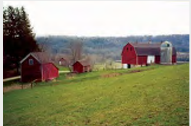
This sample application was developed for the barn on the right pictured above. The image below, left, shows a deteriorated section of the limestone foundation.
